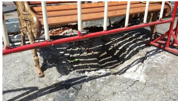
Figure 1 Damage level of RC fence column and RC slab (photos from [34] and Than Tao Mahaprom Foundation)
